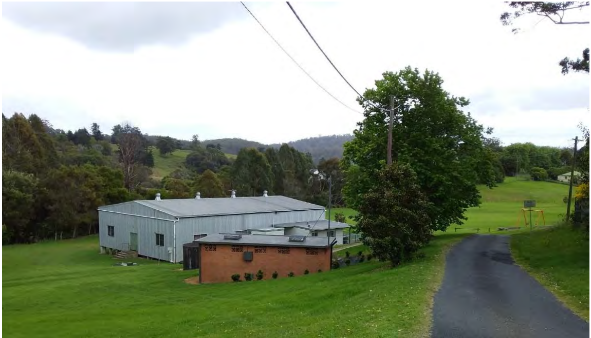
Figure 5.4.11: Street view Eastern Dorrigo Community Hall, public toilets and showground
