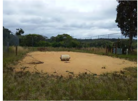
Figure 5.4.36: Tennis court in disrepair
