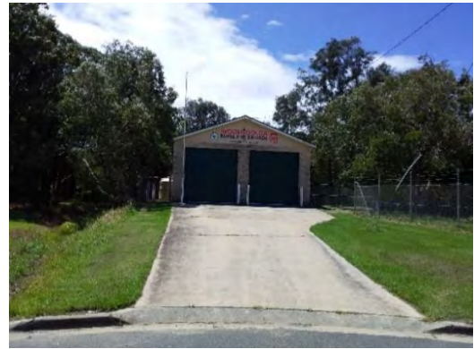
Figure 5.4.28: Woolgoolga RFS station on Ganderton Street
