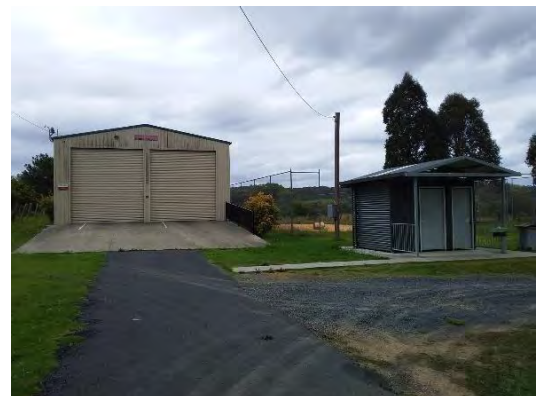
Figure 5.4.34: RFS shed and public toilets
