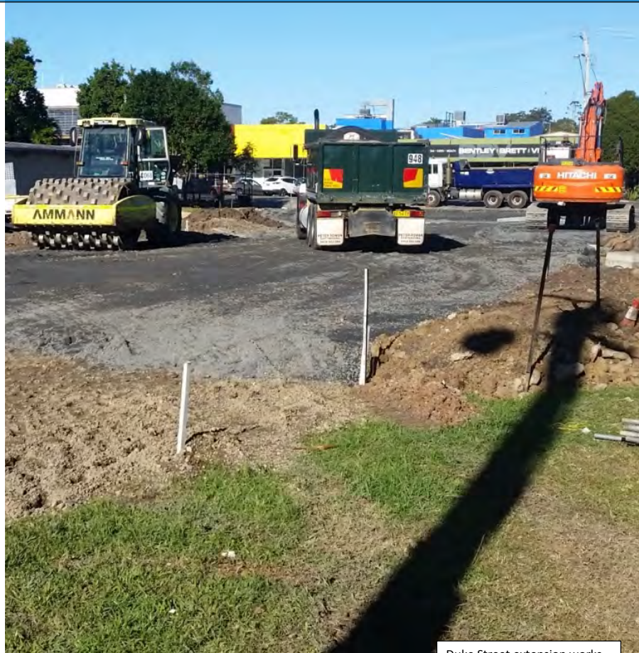
Duke Street extension works
