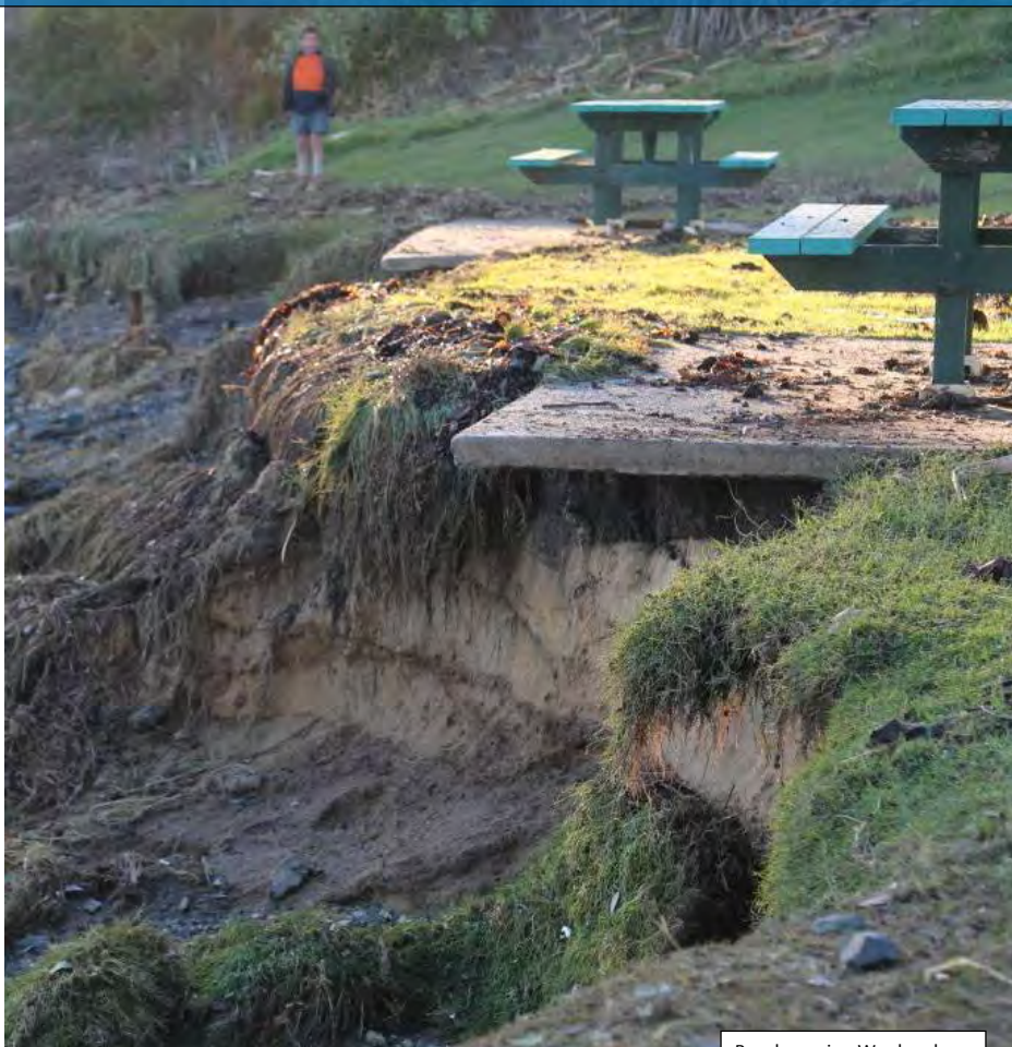
Beach erosion Woolgoolga
