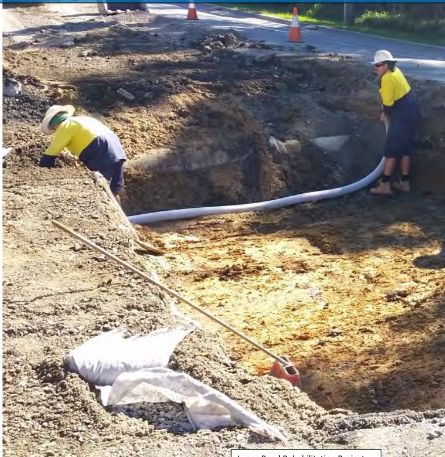
Lyons Road Rehabilitation Project
