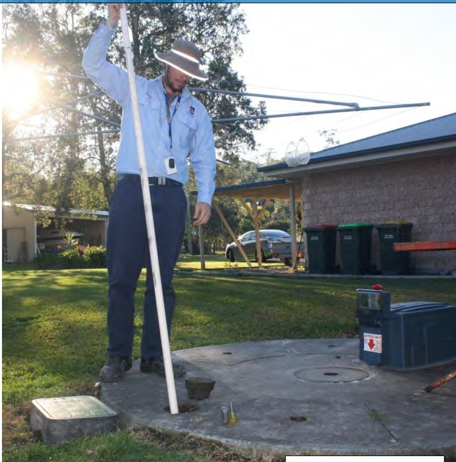
Onsite Sewage System Management
