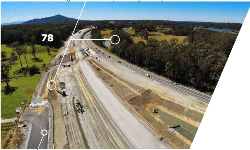
Pacific Highway upgrade, Valla
