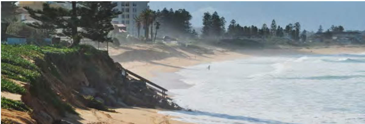
Erosion at Collaroy-Narabeen beach (Angus Gordon)
