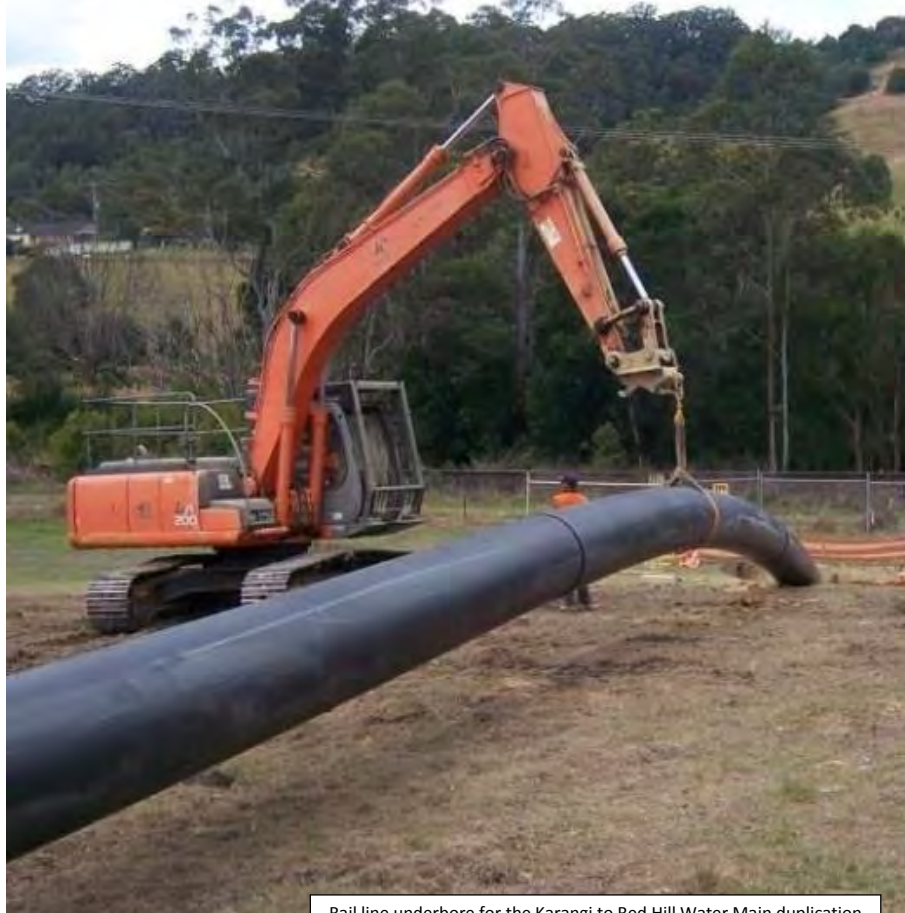
Rail line underbore for the Karangi to Red Hill Water Main duplication
