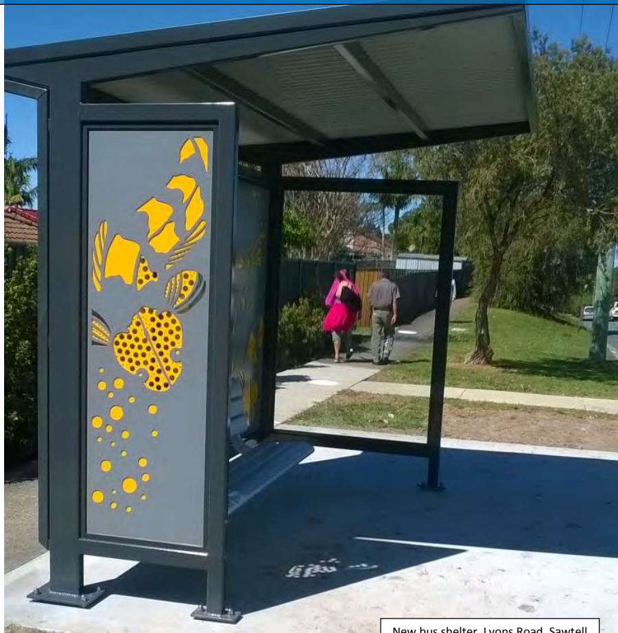
New bus shelter, Lyons Road, Sawtell
