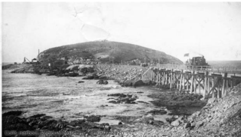
Plate 1. c1915 timber trestle bridge and rail line built to access the quarry on South Coff Island, 1915 – 1928 (Source: Hedditch, 2012:5)
