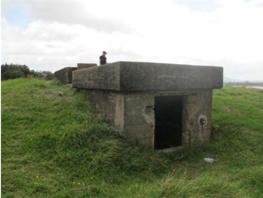
Plate 4. Front compartment of the heritage item.
