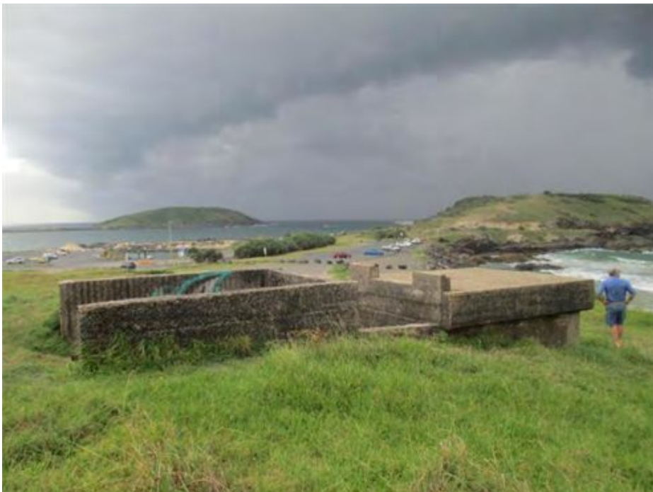
Plate 3. Heritage item on Bunker headland, looking north.
