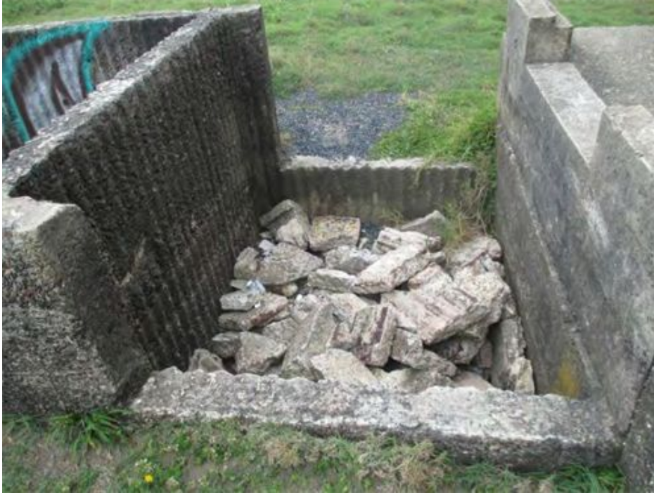
Plate 12. Middle compartment with rubble, presumably from the former roof. Note: opening on both sides of the item.
