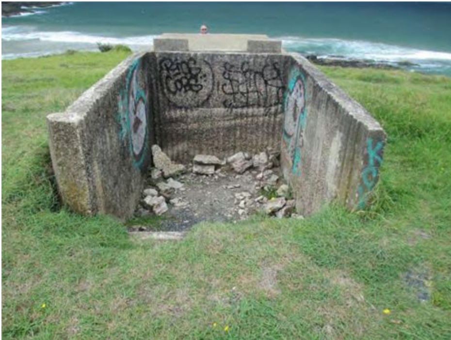
Plate 13. Rear compartment of the heritage item, with opening at rear and at least two steps leading down to concrete floor. Note: the frequent graffiti.
