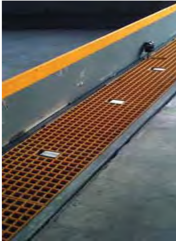
Figure 7-6 Permanent Automatic 'Flip up' Flood Barrier (source: http://www.spec-net.com.au/press/0212/flo_150212.htm )
