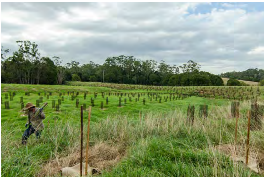
Revegetation works in the Orara Valley
