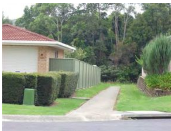
Plate D1.3 Path to nowhere. This pedestrian corridor leads into a hidden area of drainage reserve that offers minimal recreational value and poor passive surveillance
