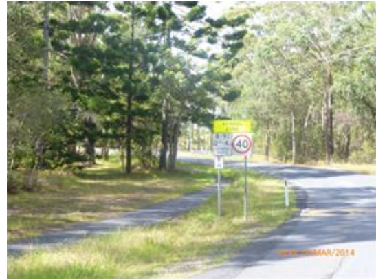
Arrawarra Road off- road cycleway
