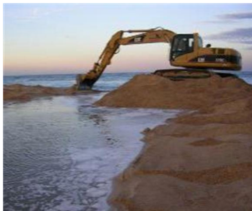
Image: Artificial opening of Burrill Lake. Photo by R. Massie Source: NSW Government (undated)
