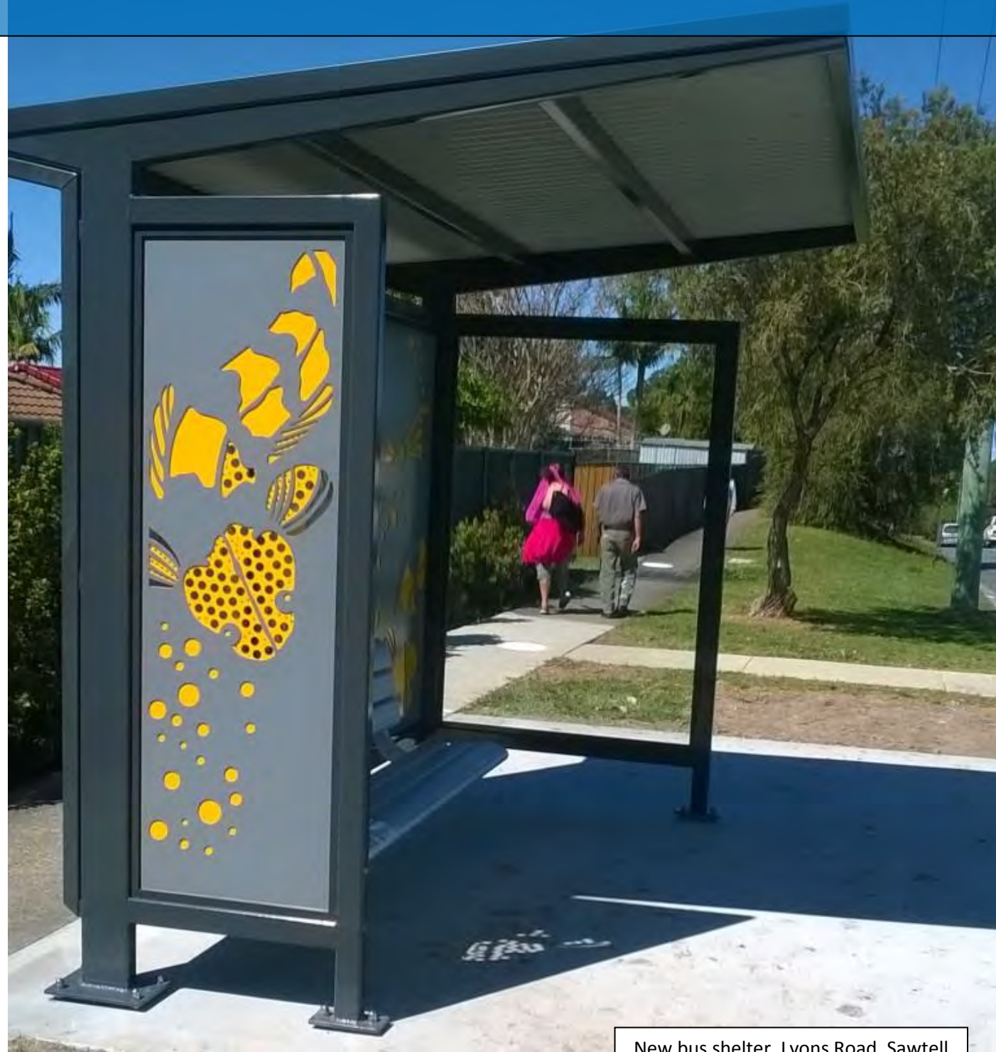
New bus shelter, Lyons Road, Sawtell
