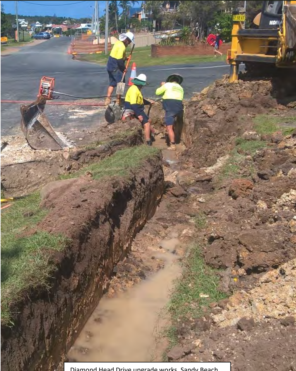
Diamond Head Drive upgrade works, Sandy Beach.
