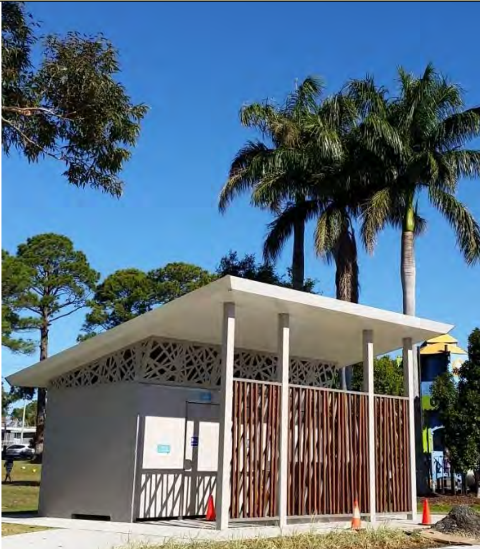
A new public amenities building was installed as part of the redevelopment of Brelsford Park.
