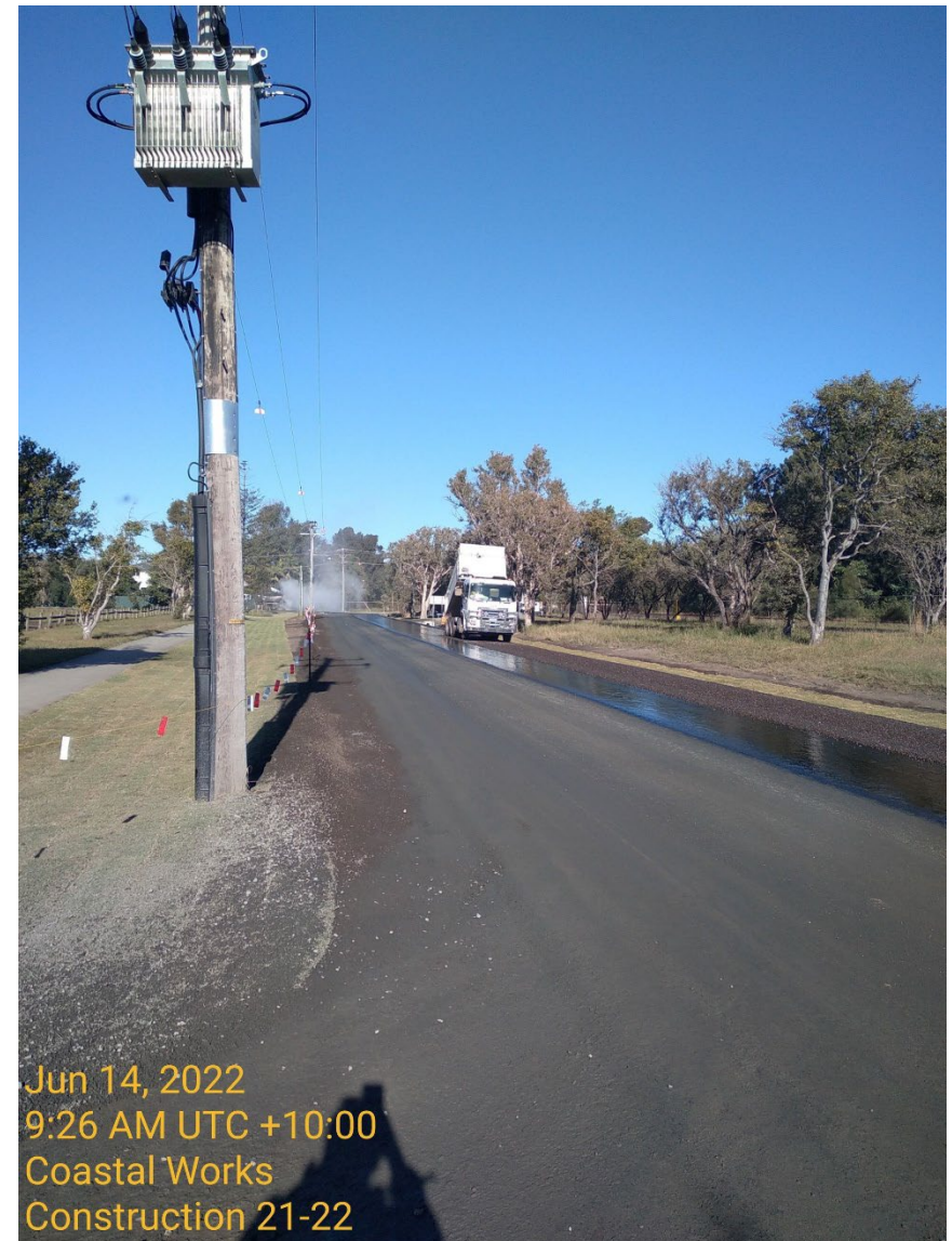
Above: Construction works on Hulberts Road
