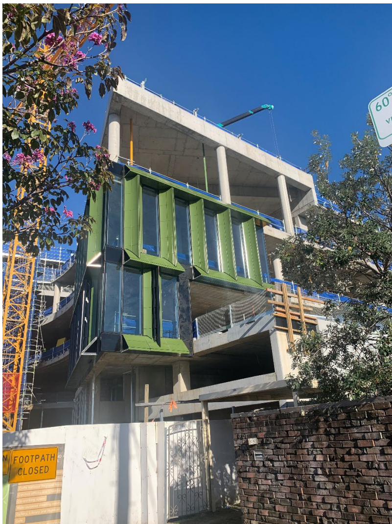
Above: Yarrila Place, building progress.
