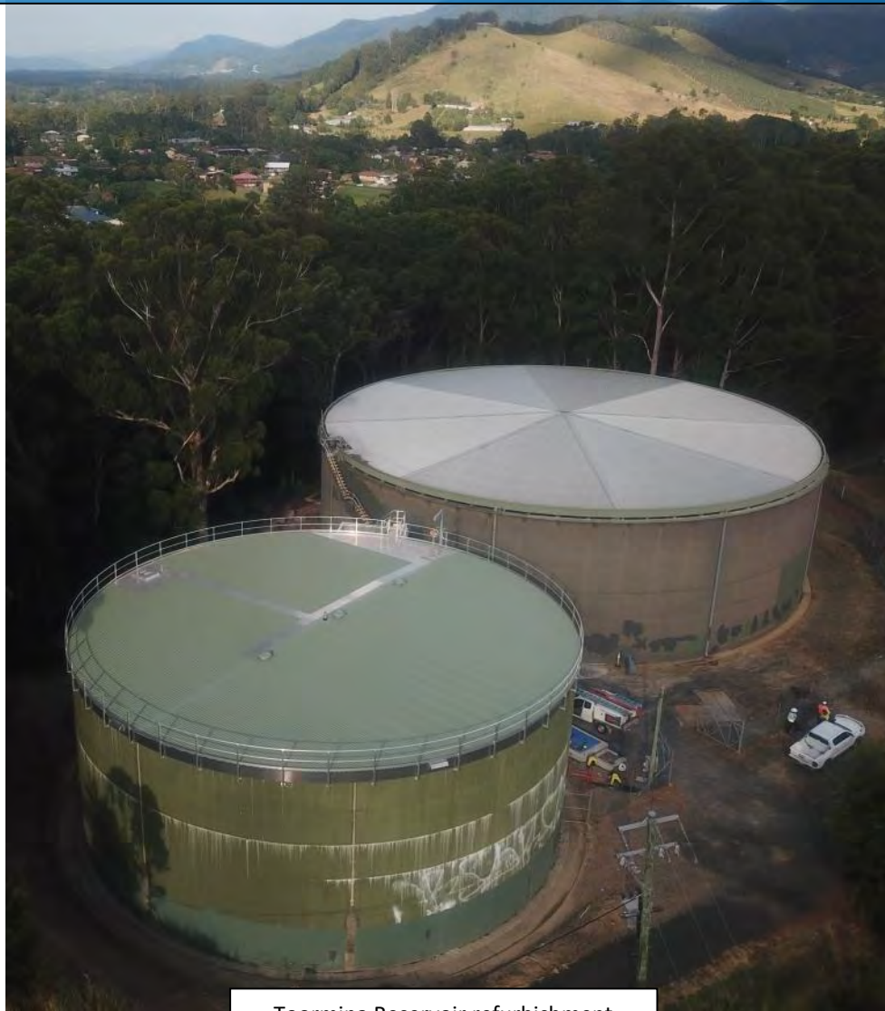
Toormina Reservoir refurbishment
