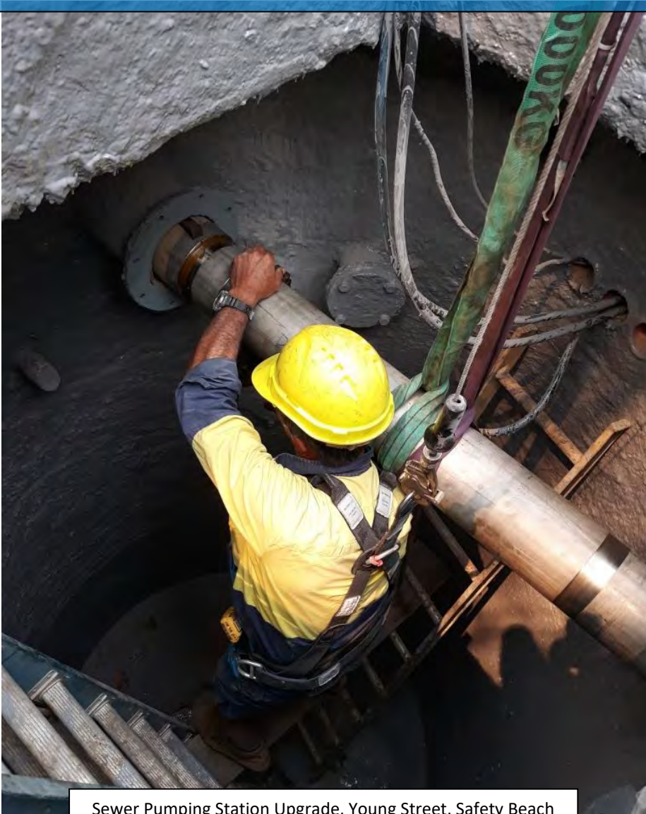
Sewer Pumping Station Upgrade, Young Street, Safety Beach
