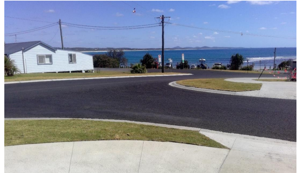
2 nd and 3 rd Avenue road renewal at Arrawarra
