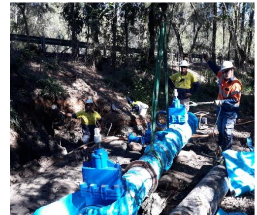
Water main installation at Sawtell Rd, Boambee Creek Bridge
