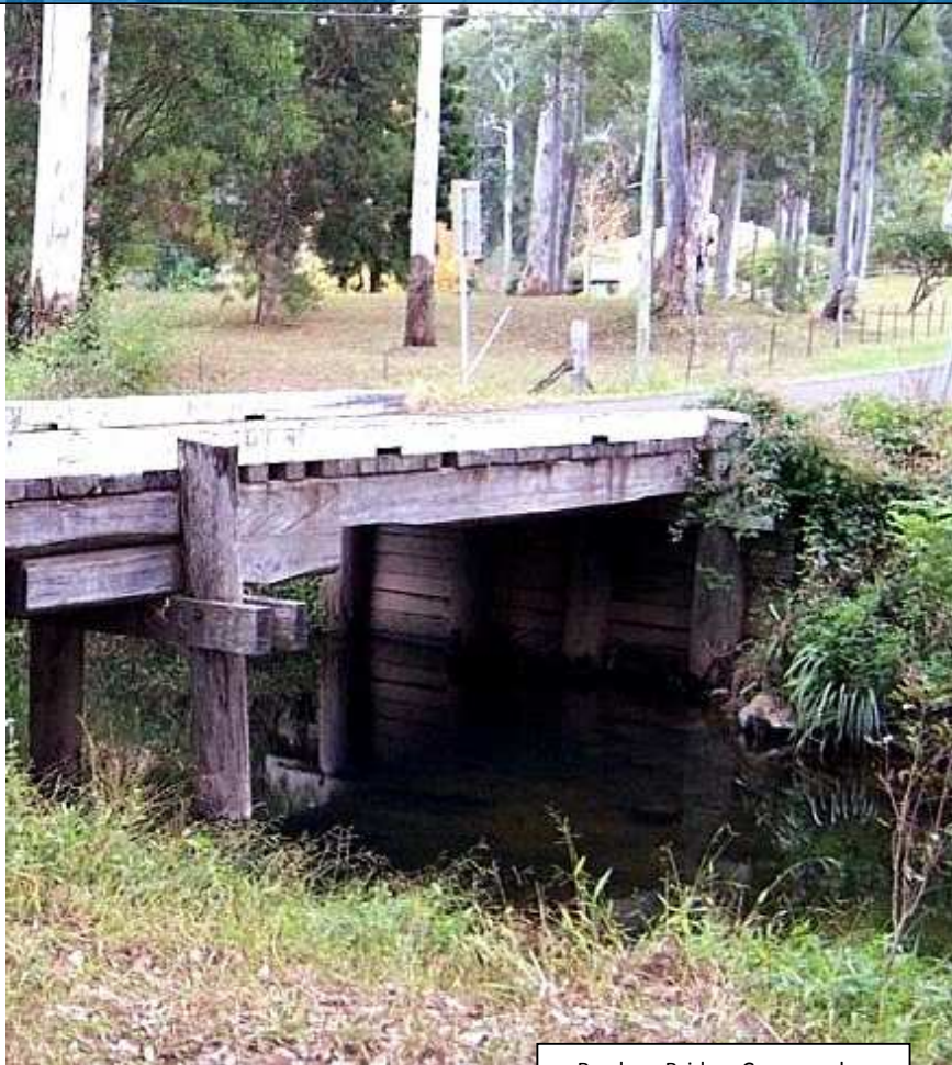
Bardens Bridge, Crossmaglen
