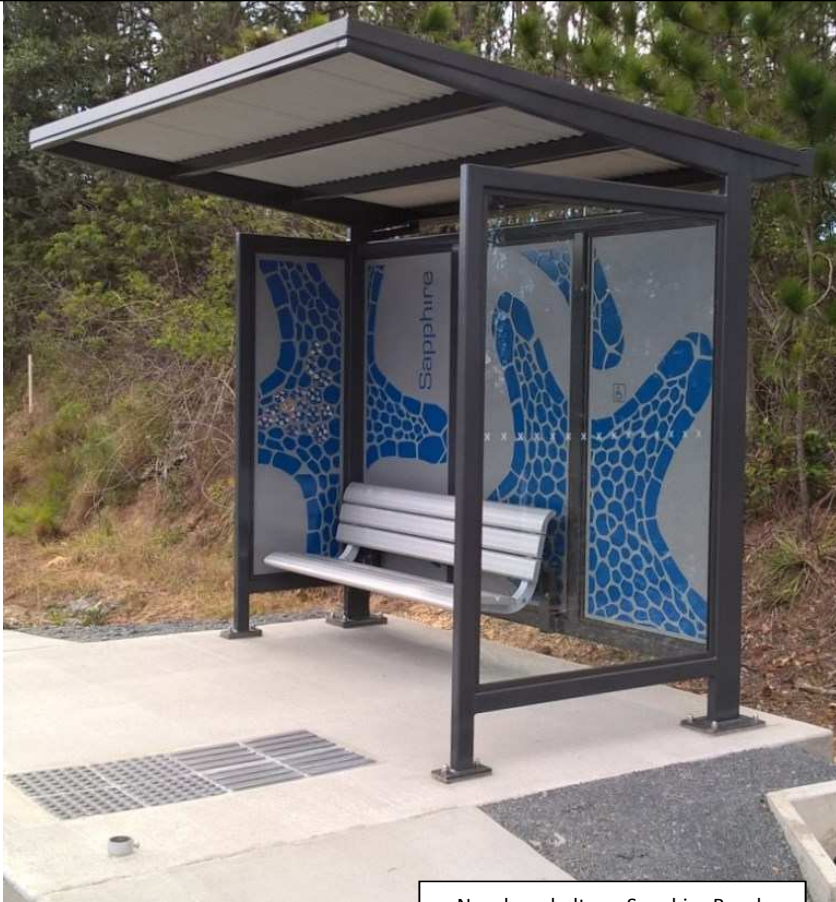
New bus shelter – Sapphire Beach
