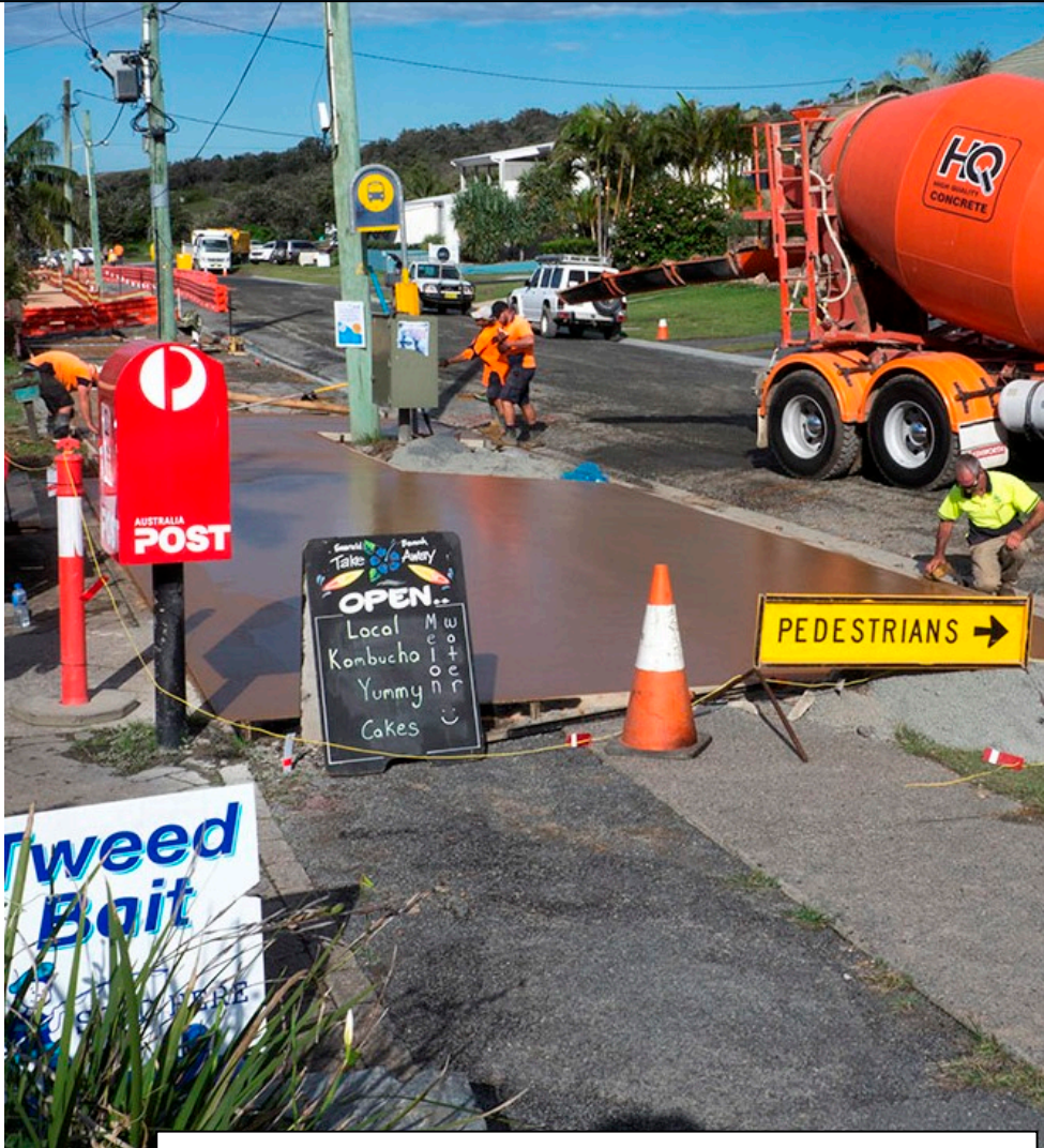
Construction of a shared footpath/cycleway on Fiddaman Road, Emerald Beach.
