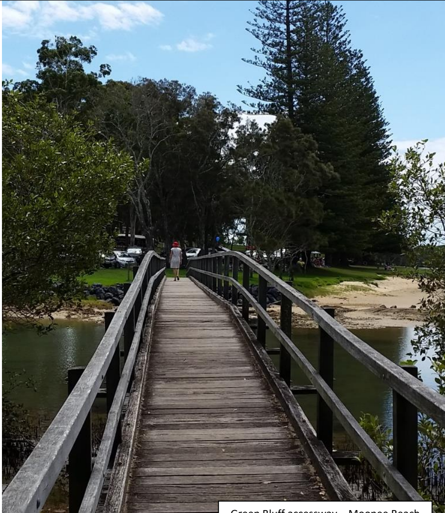
Green Bluff accessway – Moonee Beach
