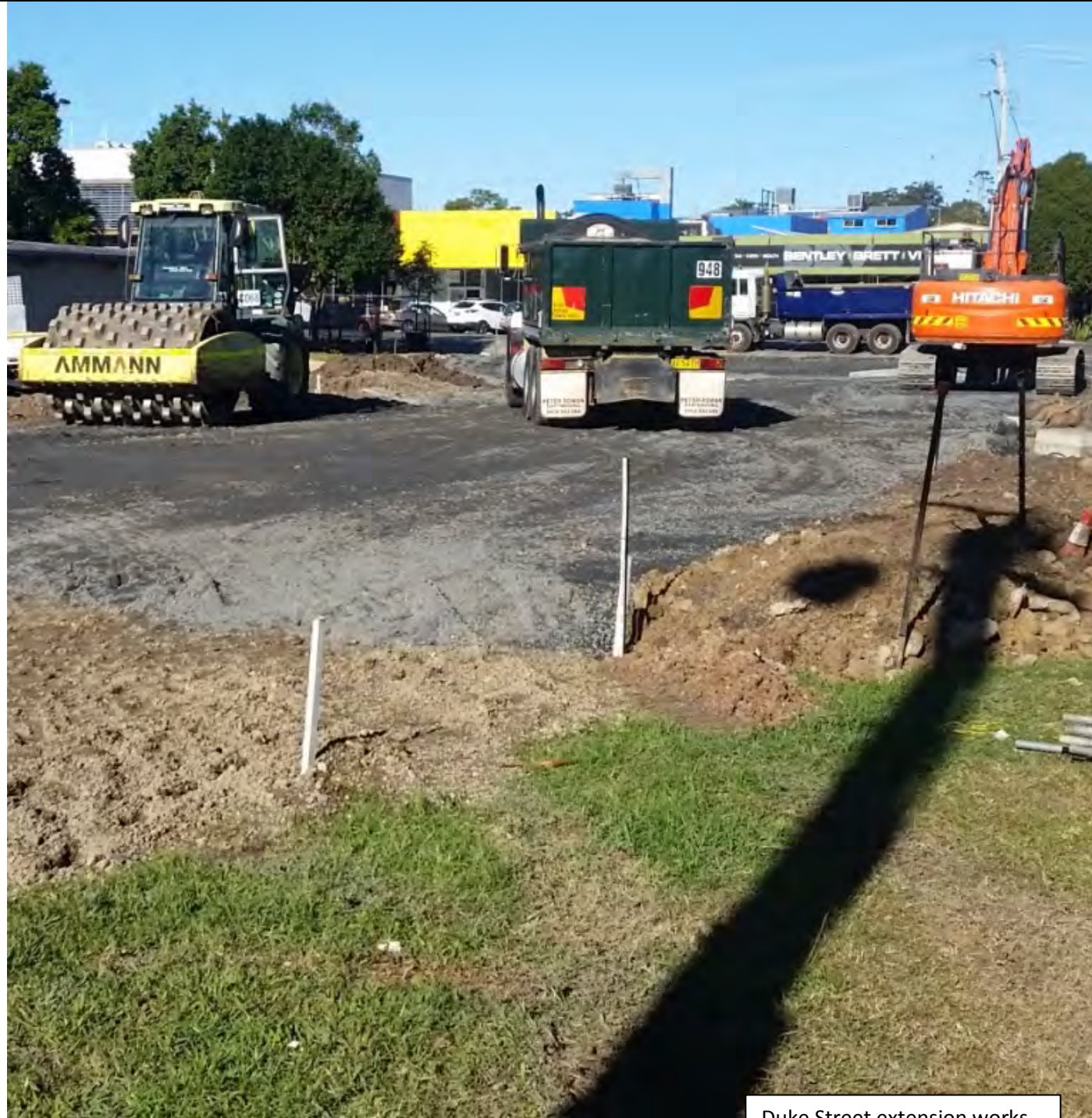
Duke Street extension works
