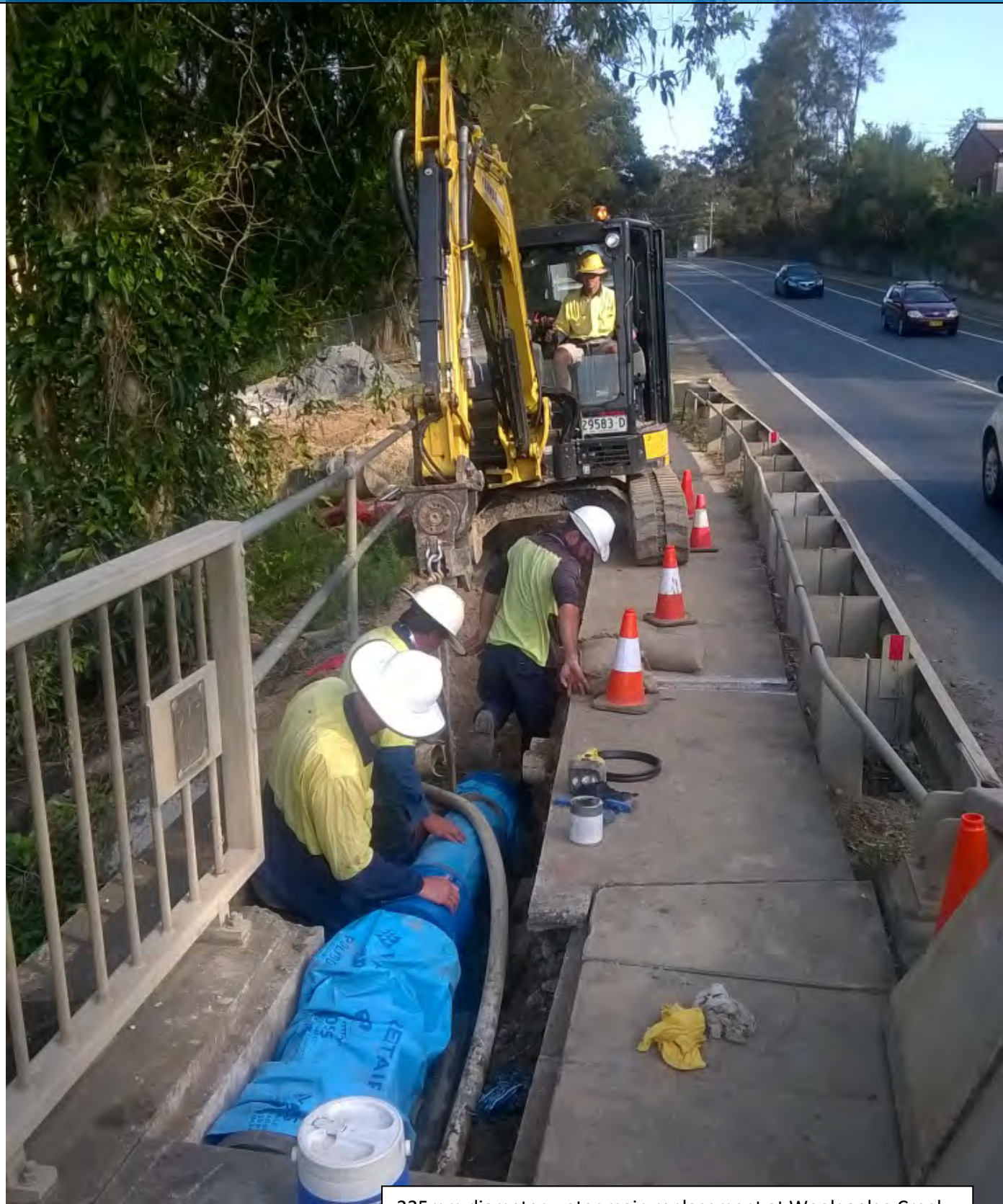
225mm diameter water main replacement at Woolgoolga Creek
