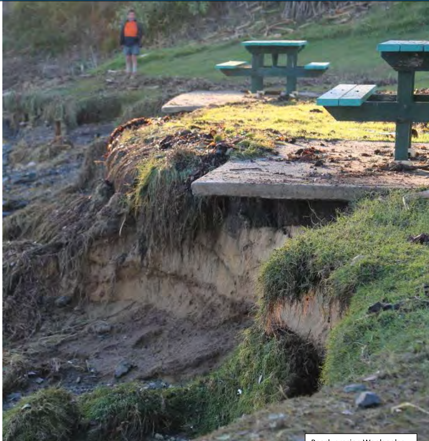
Beach erosion Woolgoolga
