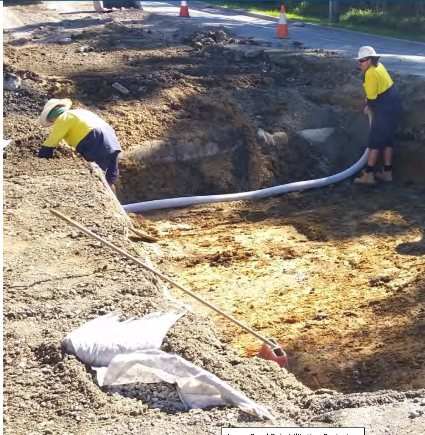
Lyons Road Rehabilitation Project
