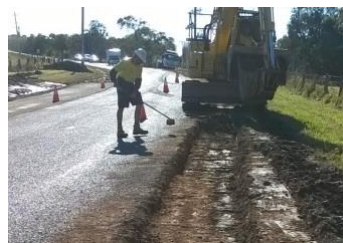
Red Rock cycleway construction
