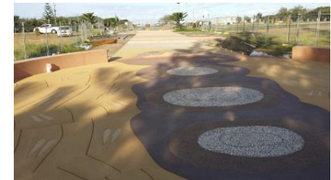
New Jetty Foreshore walkway
