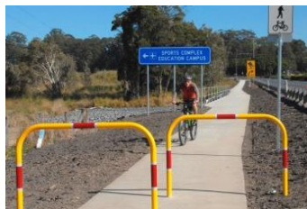
South Coffs Cycleway
