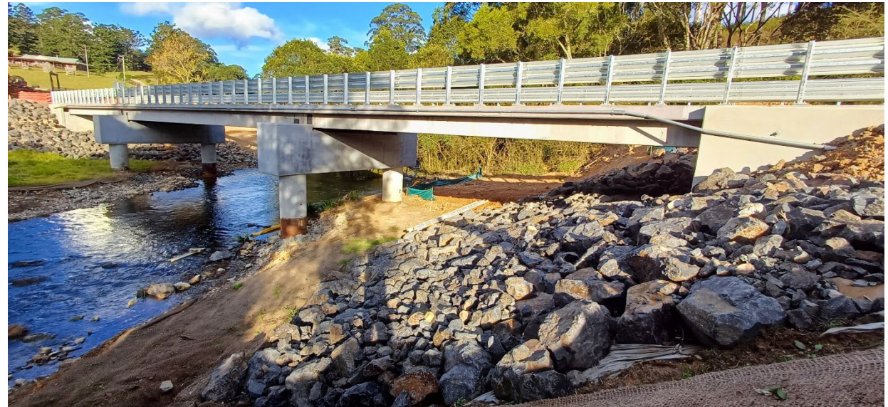
Bobo Bridge works
