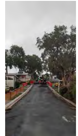
Below: Wet weather damage checks and repair, March, 2021
