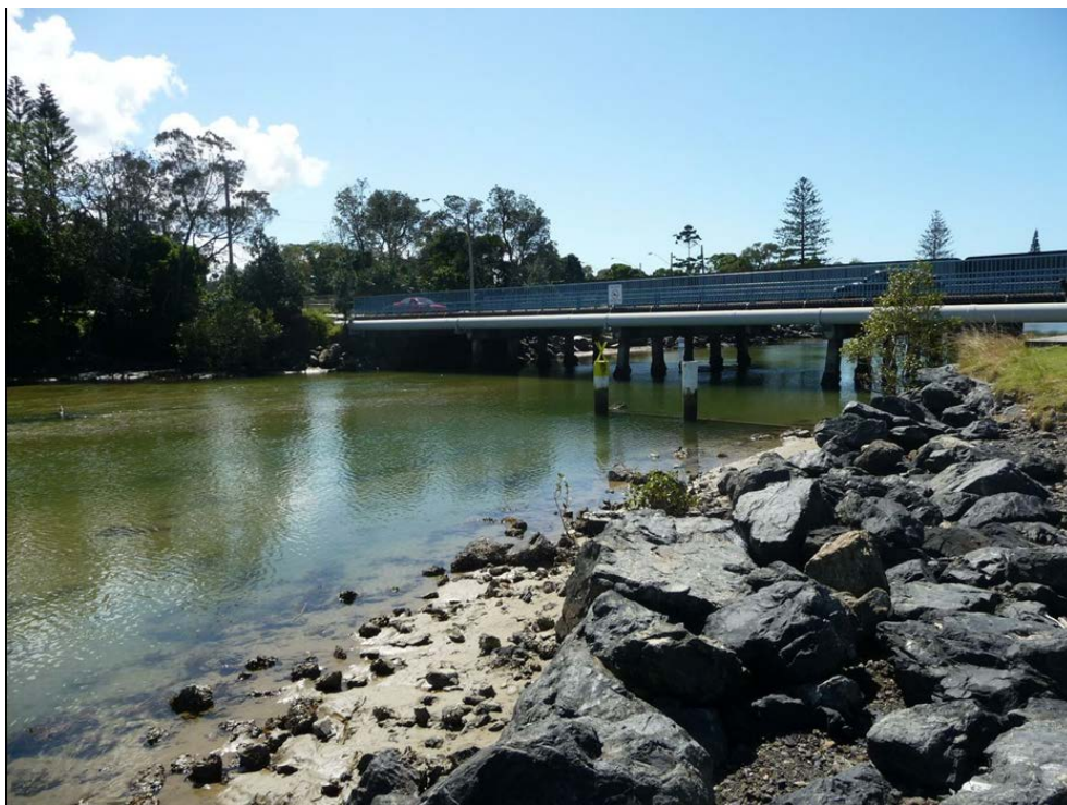
Figure 3.3.3 Site COFFS1 in Coffs Creek looking downstream from crossing.
