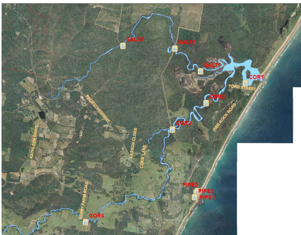
Figure 3.9.1 Dominant land-use and location of sites on Corindi River and Saltwater Creek in the Coffs Harbour catchment (Source CHCC).
