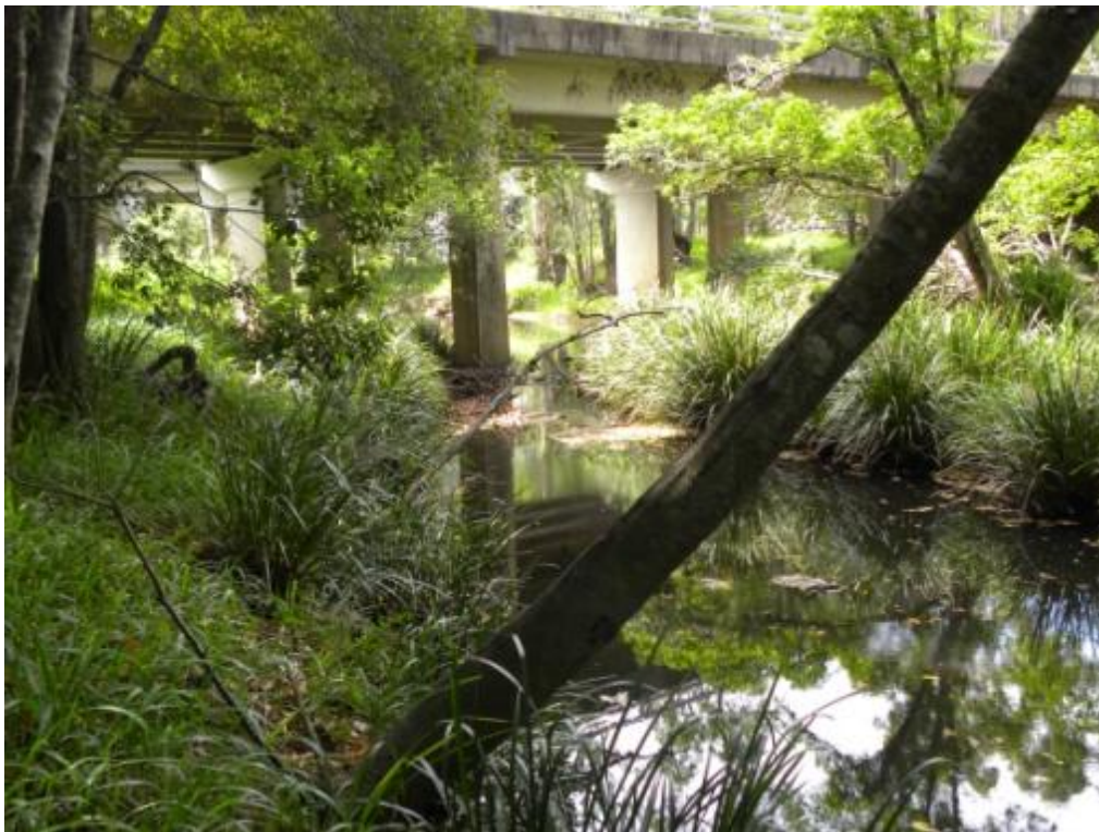
Figure 3.1.2a Site PINE3 in Pine Creek looking downstream from crossing.
