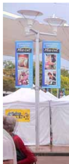
Existing Pole Top Light Pole
