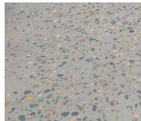
Exposed aggregate concrete path Broom finish to edges
