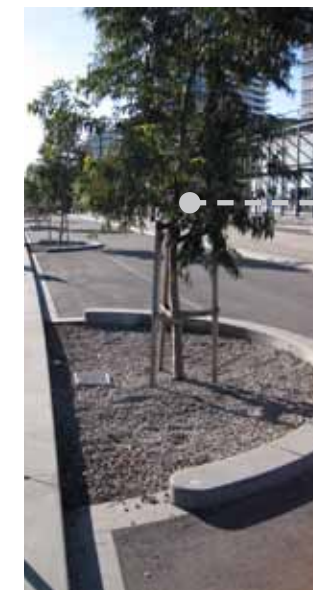
Example Trees in roadway with water sensitive urban design
