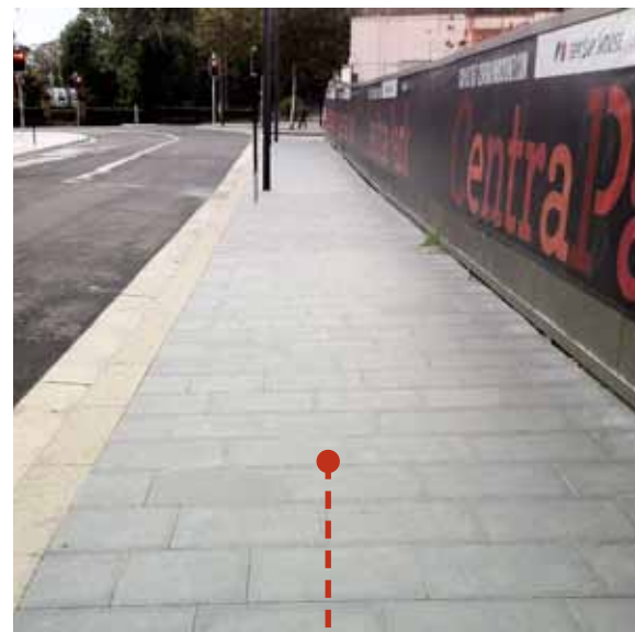
Example of simplified palette with large format paver with no banding and 300mm wide Kerbs
