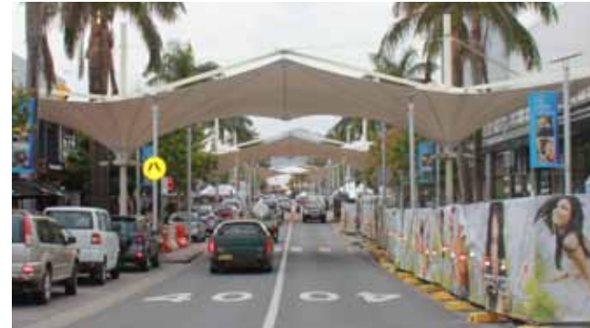
Existing Shade Sails to Harbour Drive
