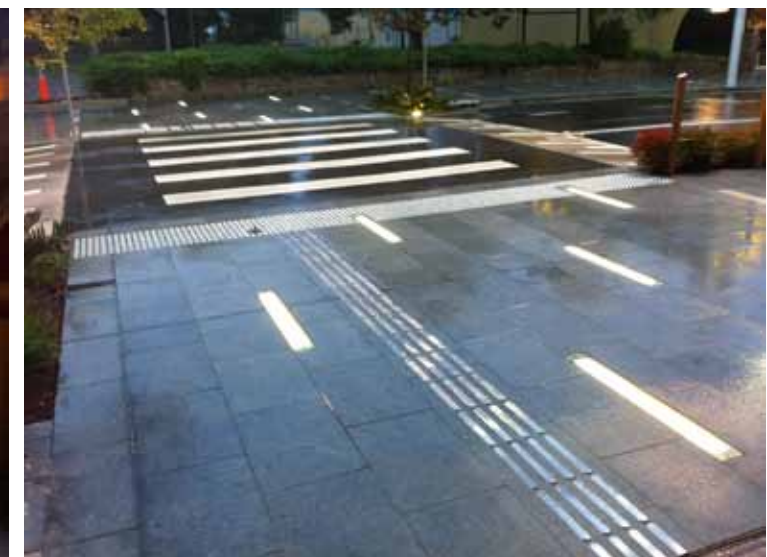
Feature Lighting in pavement to crossings adjacent City Square
