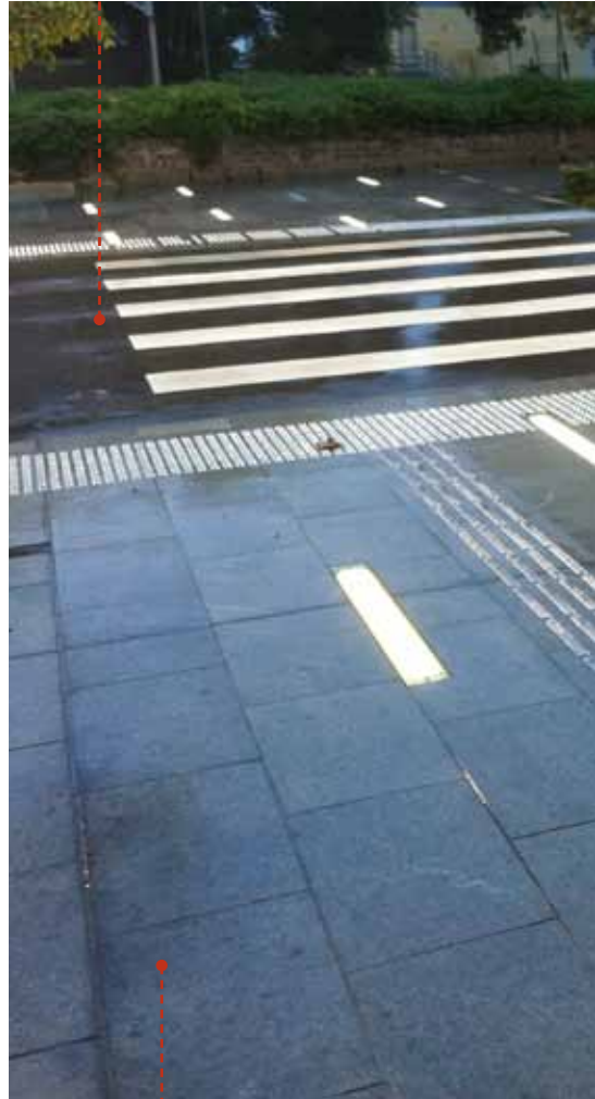
City Centre Main Street Granite Pavement 'Sesame Grey' (Wet)
