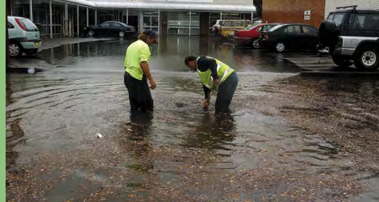
Inadequate drains in Park Avenue
