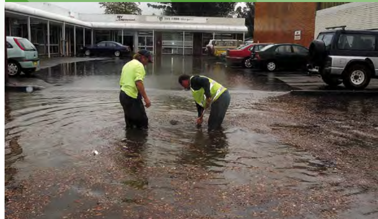
Location: Council workers unblock drains following heavy rainfall
