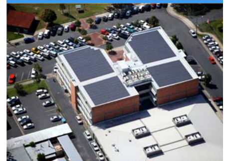
Solar Array on Rigby House rooftop
