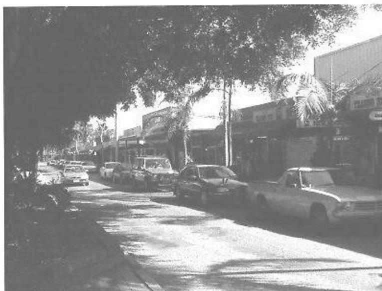
Figure 2 Photograph of First Avenue, Sawtell
